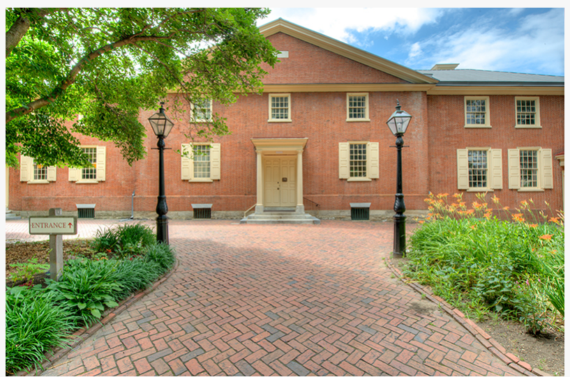
Exterior of Arch Street Meeting House
