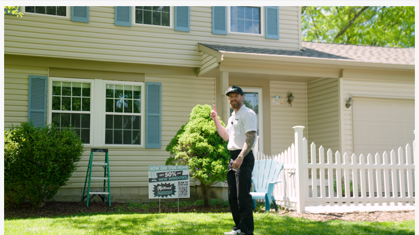
Post Window Installation by (McCloud Windows) in Pittsburgh, PA
