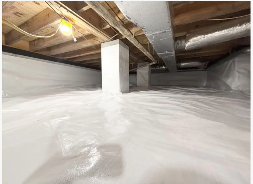
Full Crawlspace Encapsulation
