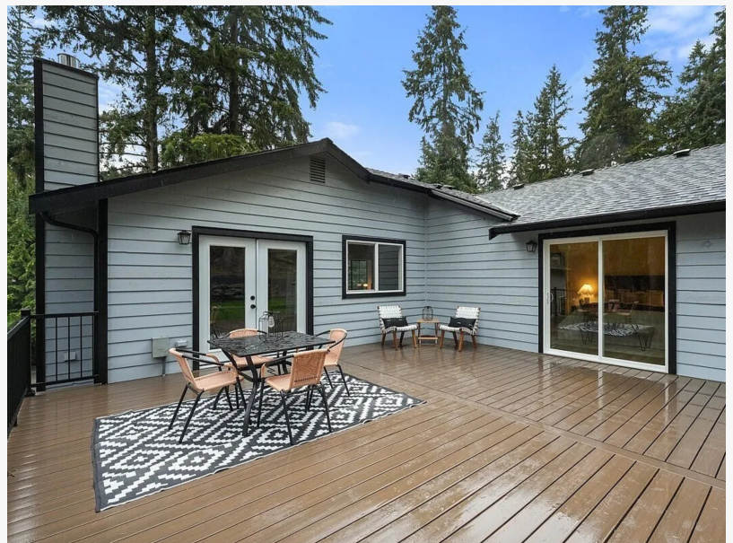
Deck Renovation After
