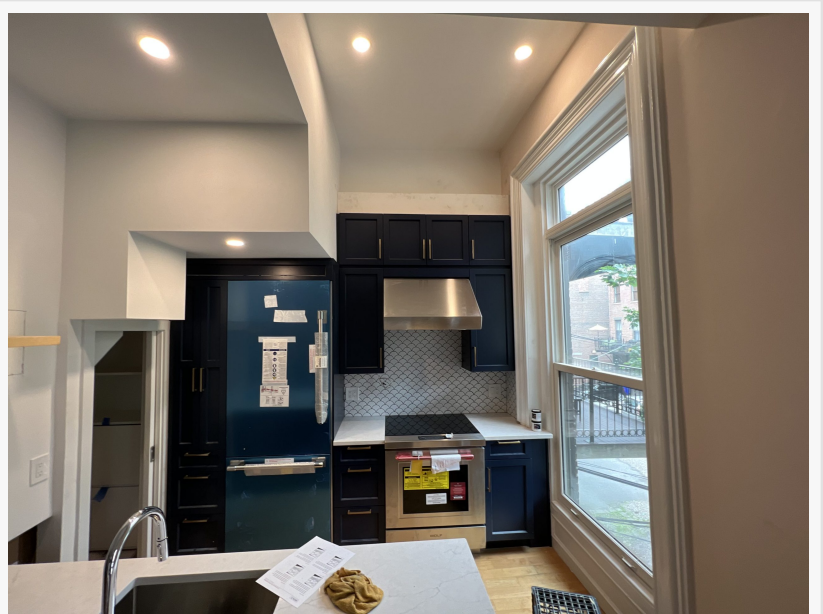
kitchen remodeling in South End
