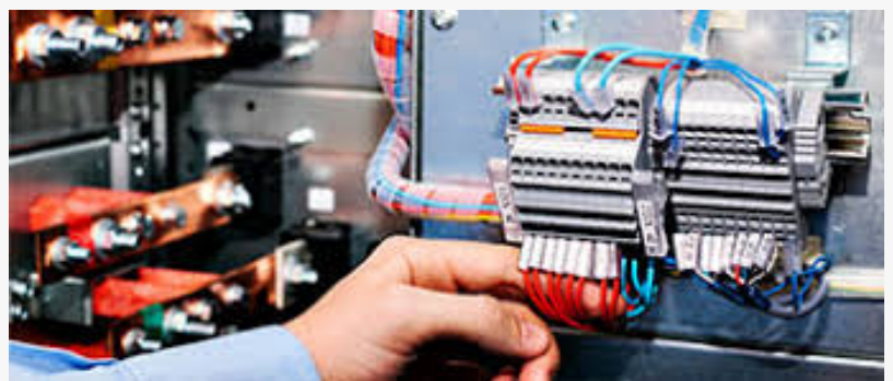
Electrical Estimating Services
