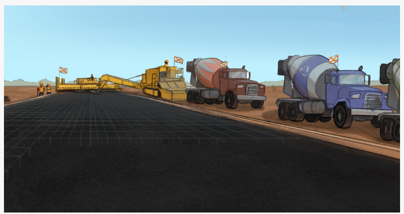
After completing the design, the concrete paving crew places rebar and begins pouring the new runway
