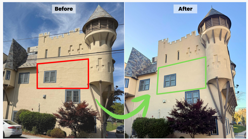
Before and After Stucco Wall Repair
