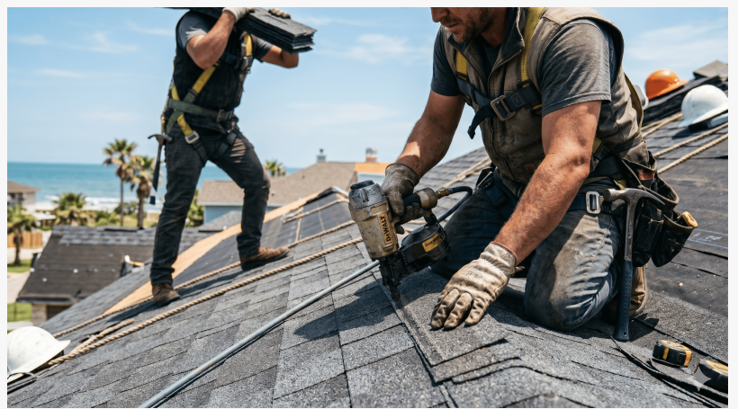
Roof Repair in Corpus Christi, TX
