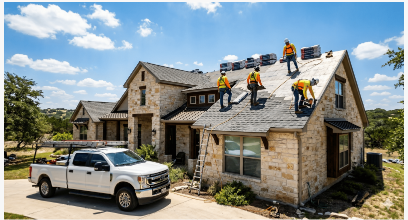
Roofing Contractor in San Antonio, TX
