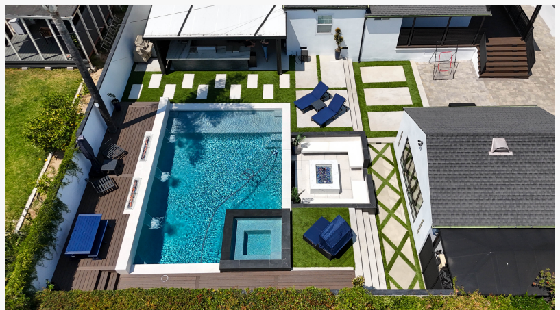
Complete Backyard Renovation by Exodus Construction
