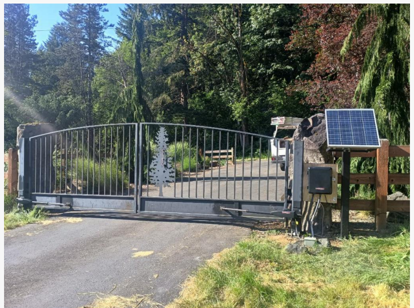
Farm style HOA gate installation - first impression
