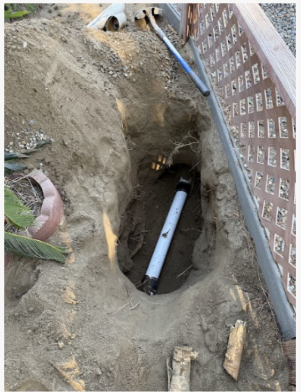
Expert excavation and sewer repair to maintain your home's vital underground systems.
