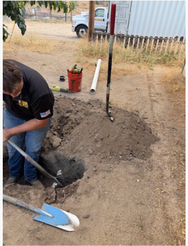
Expert excavation and sewer repair to maintain your property's essential infrastructure.
