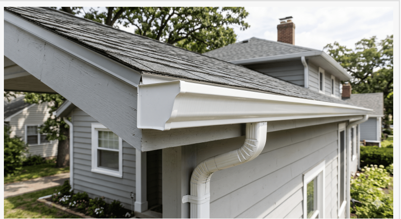
Gutter Installation in Eustis, FL
