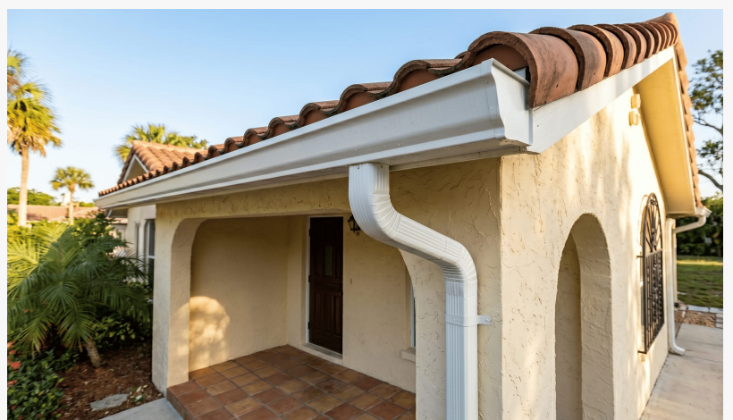
Seamless Gutter Installation in High Springs, FL
