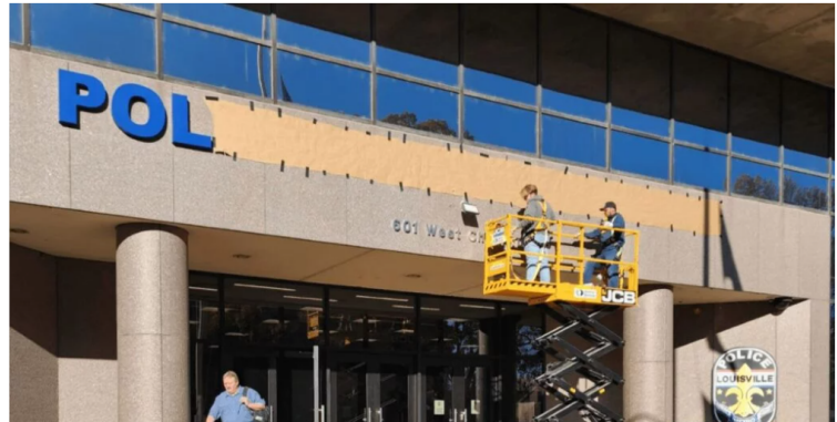
Installation of dimensional building letters at the main entrance of Louisville Metro Police Headquarters.
