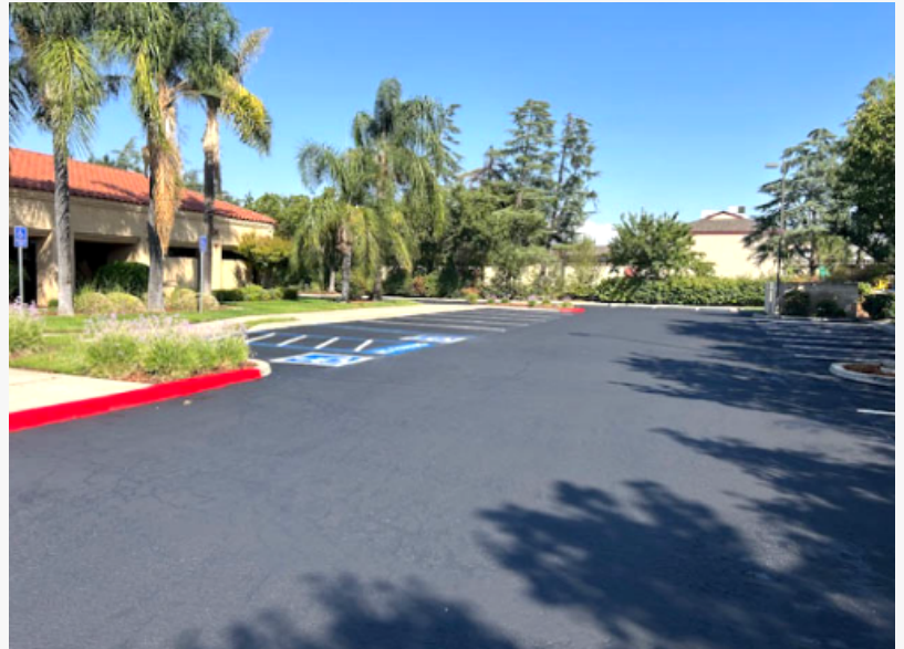
Recently completed commercial parking lot paving project featuring fresh asphalt and clearly marked ADA-compliant parking spaces.
