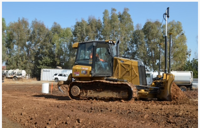
A heavy-duty bulldozer equipped with GPS-guided machine control technology, ensuring precision grading for optimized site preparation.
