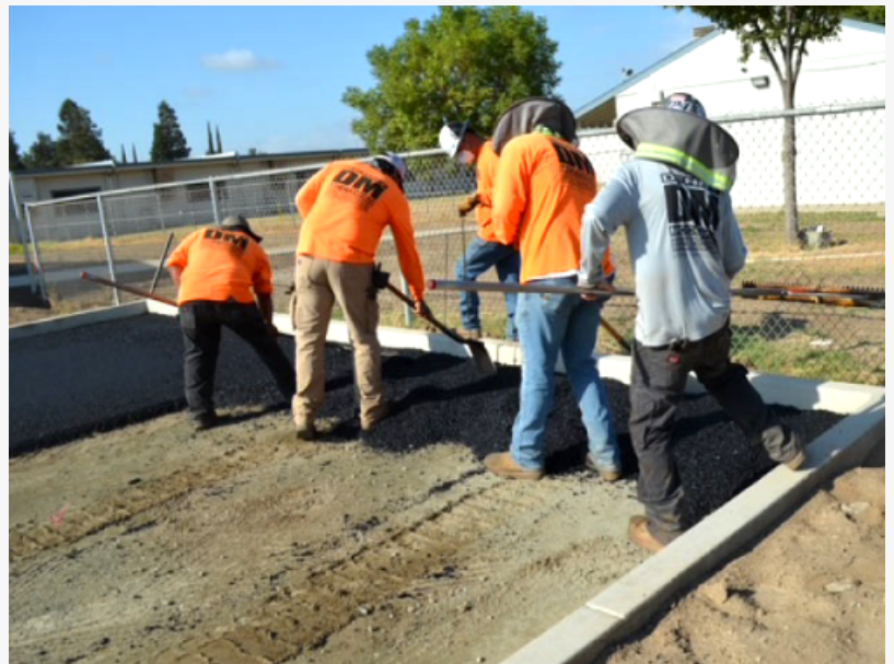
A dedicated paving crew from Denny McCowan General Engineering Inc. using manual tools to precisely distribute asphalt for a new project.
