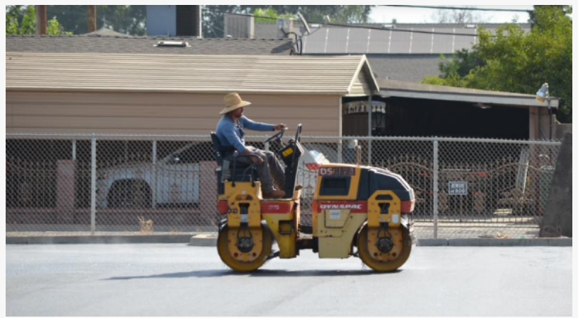
A construction professional operating a dual-drum asphalt roller to compact the surface for optimal durability.
