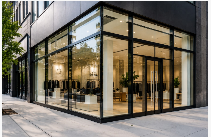
Commercial Storefront Glass Installation
