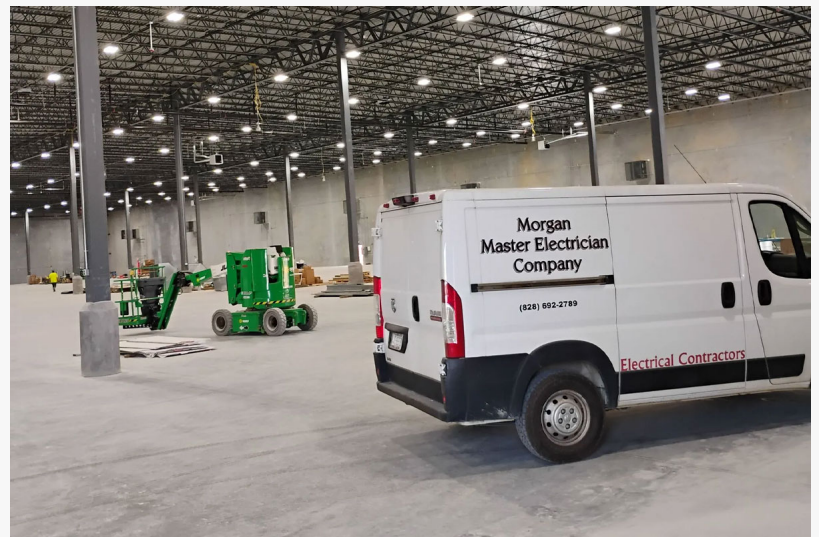
Best Industrial Electrical Services
