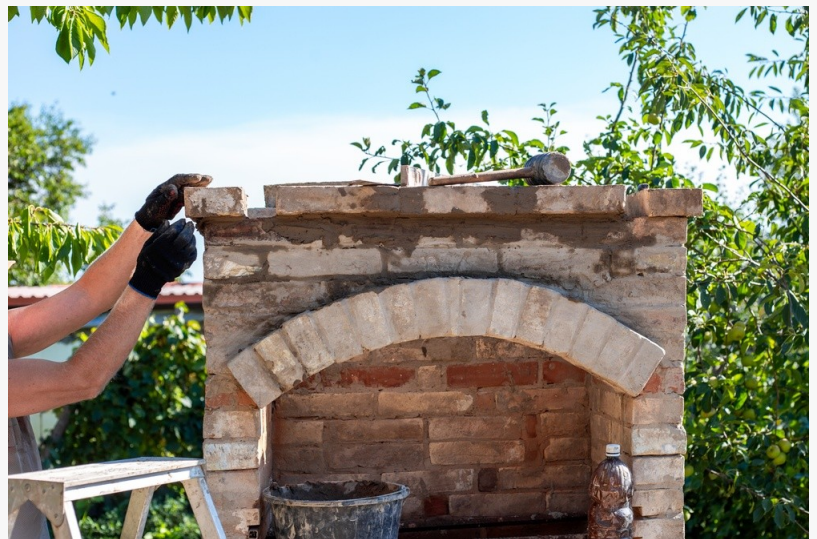
brick masonry repair in Salem
