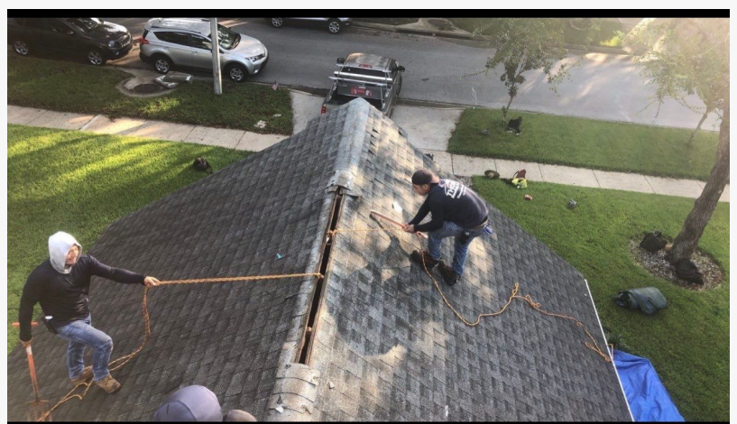
Roof Repair in Orlando, FL
