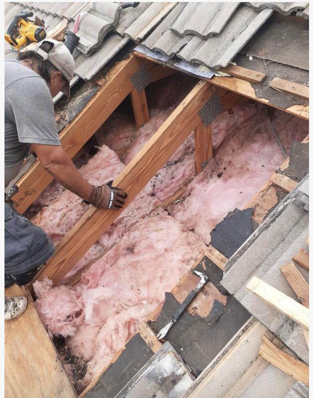
Roof Repair in Melbourne, FL
