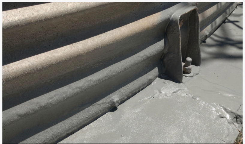
Detail of a coated grain-bin wall and floor transition after spray-applied polyurea lining.
