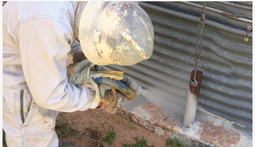
Applicator sprays a protective polyurea lining along the lower wall and floor transition of a corrugated grain bin.
