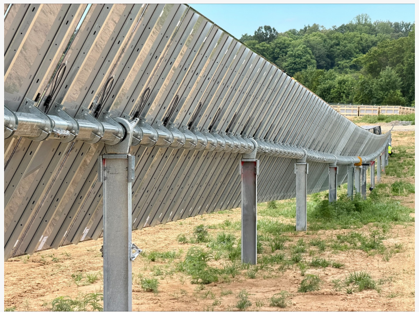
Create Energy ONTRACKER system being installed by Boyd Jones Construction at BlueStem Energy's solar site.
