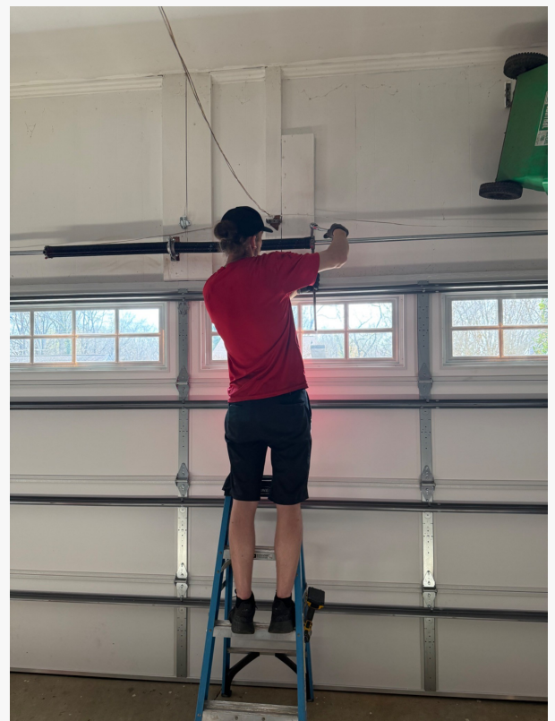
A Garage Doors Today Greenville technician performs service work on a residential garage door spring system. The locally owned company provides garage door repairs, spring replacements, tune-ups, and new door installations throughout Greenville and the su
