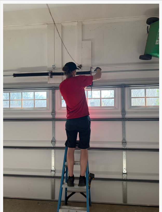
Garage Doors Today replacing a spring
