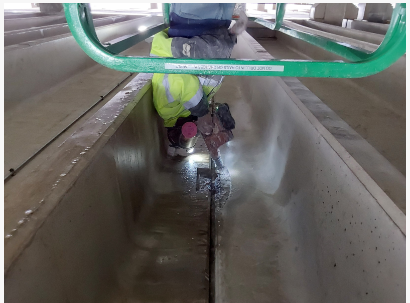
Overhead repairs on the parking garage
