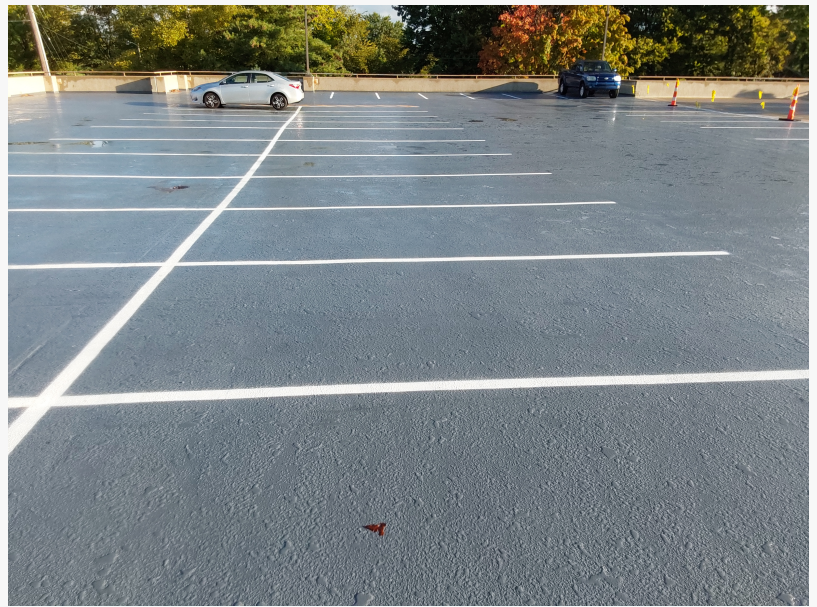
St Joseph Office Park Garage
