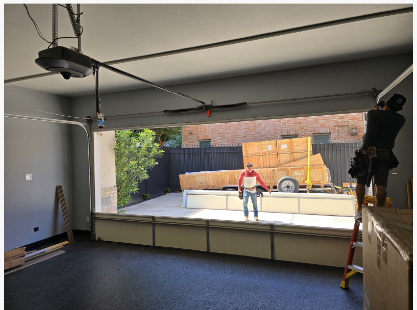
Next Hour helps reset and repair off-track garage doors throughout Santa Clarita Valley.
