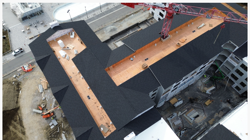
Union Square Apartments Roof
