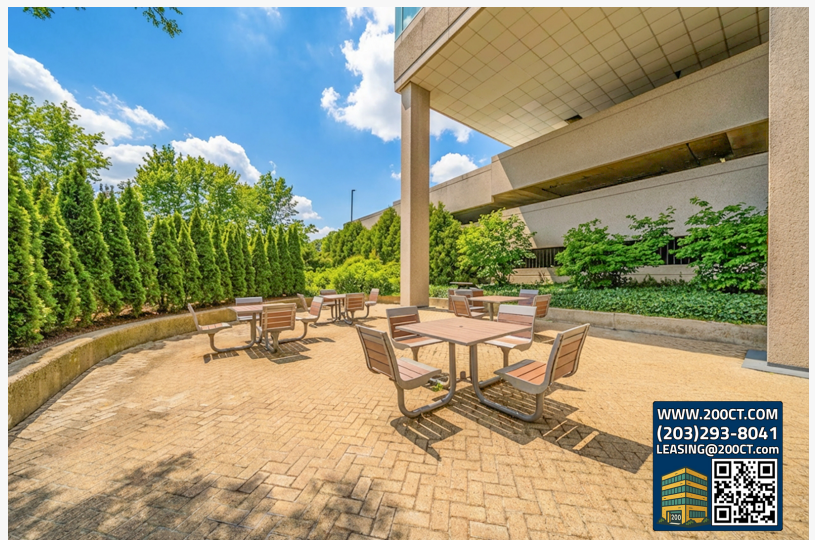
Outdoor Patio at 200 Connecticut Avenue Building Upgrades 2026
