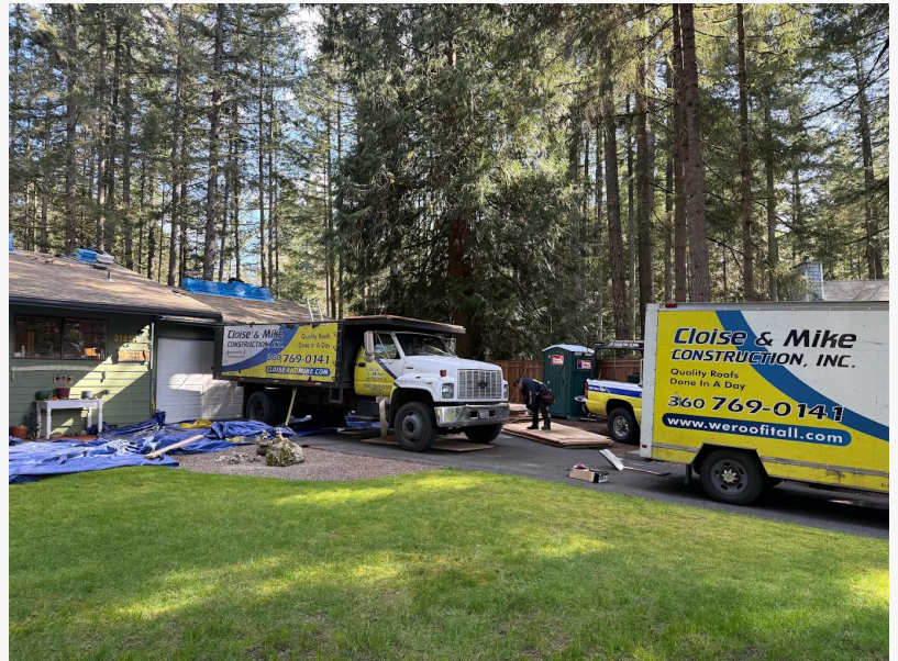
Cloise & Mike Construction Inc. crews work on a residential roofing project in Kitsap County as the company celebrates 25 years in business.
