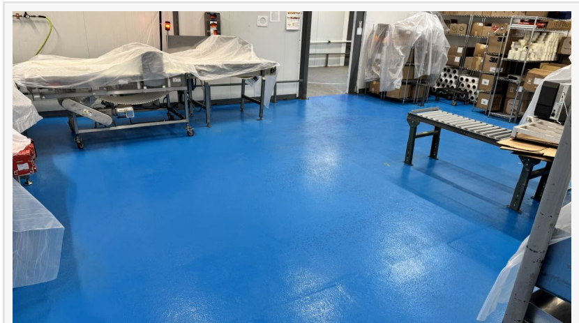
USDA Compliant Commercial Kitchen Flooring
