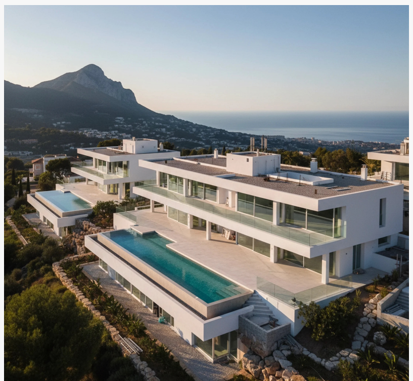
Contemporary luxury development under construction on Marbella hillside showing premium residential architecture with Mediterranean sea views
