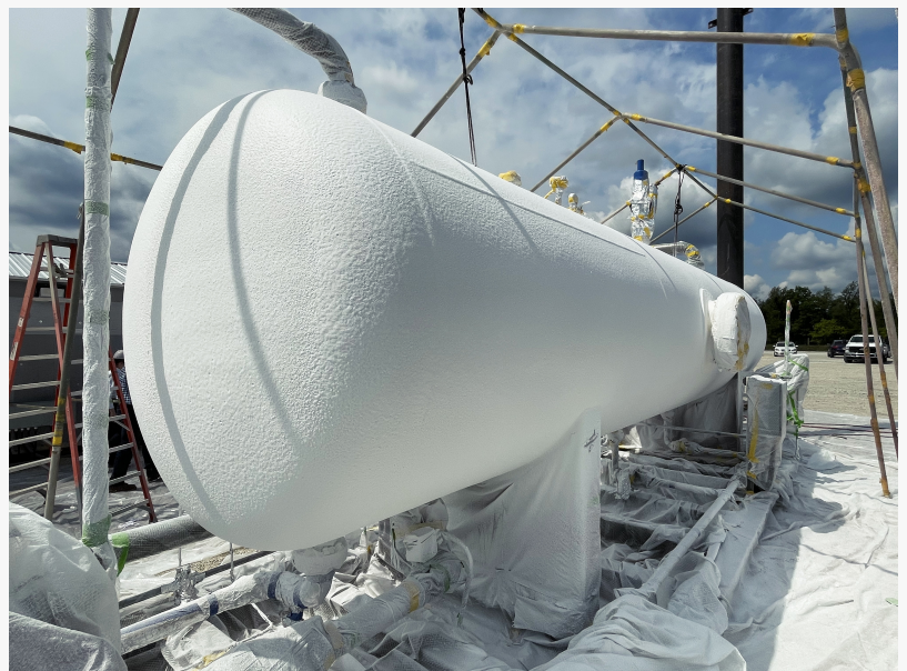
A heater treater coated with Sherwin-Williams Heat-Flex® AEB - a sprayed thermal insulative coating that replaces traditional insulation to prevent corrosion under insulation (CUI) on hot process assets.
