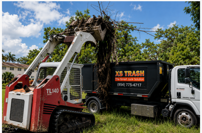
XS Trash bobcat equipment removing heavy debris during a large property cleanout project
