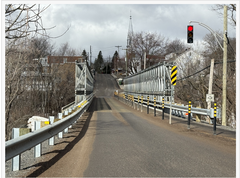
Acrow Bridge - Brownsburg Chatham - Quebec
