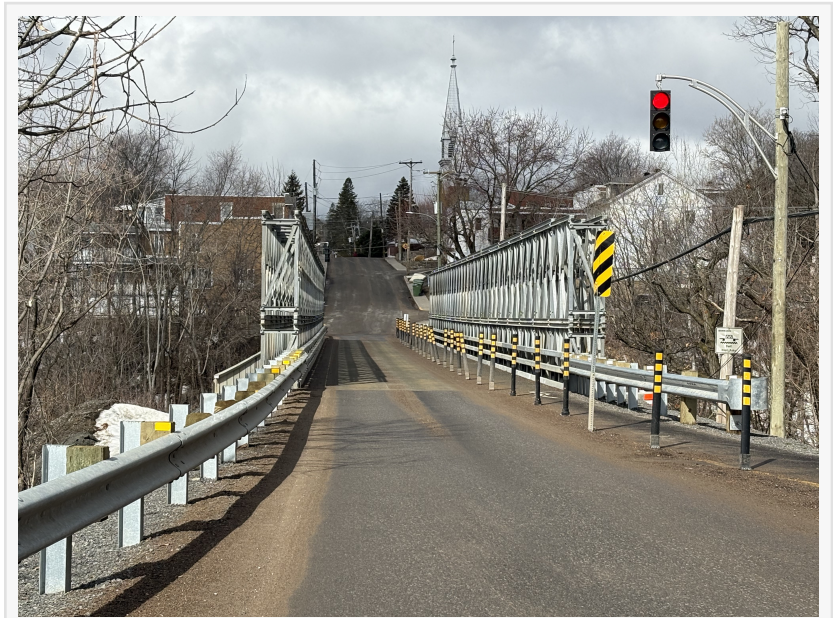
Acrow Bridge - Brownsburg Chatham - Quebec
