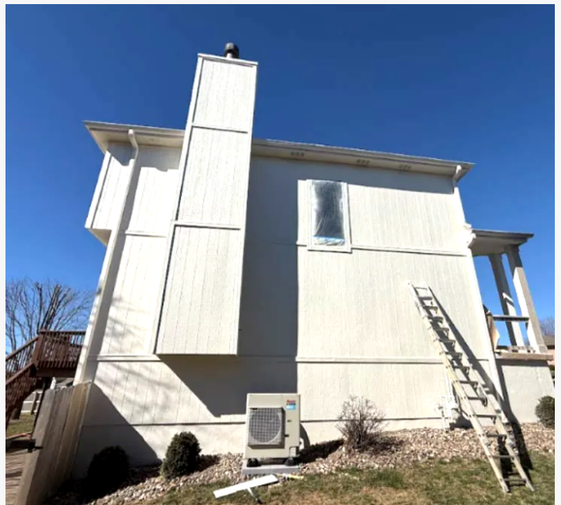
A residential exterior featuring a fresh, climate-resilient paint application, highlighting professional prep work and property protection.
