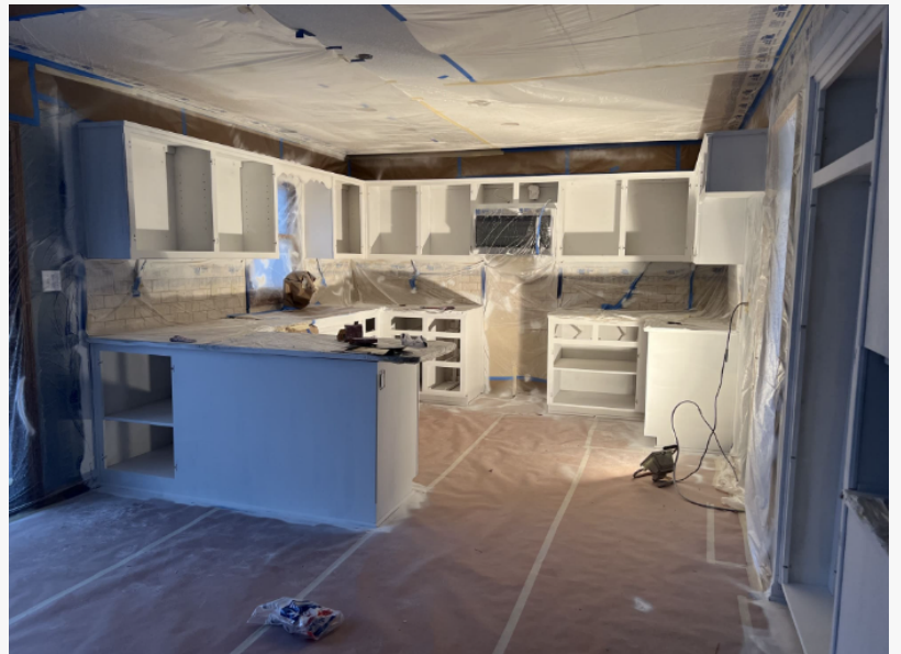
A kitchen undergoing professional cabinet refinishing, showcasing the meticulous protection of surfaces and the disciplined environment Elite77 Painters maintains during restoration projects.
