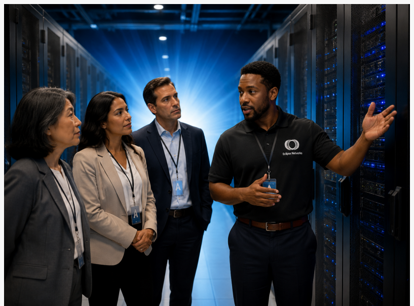
Eclipse Networks gives clients an inside look at the private cloud data center powering their technology.
