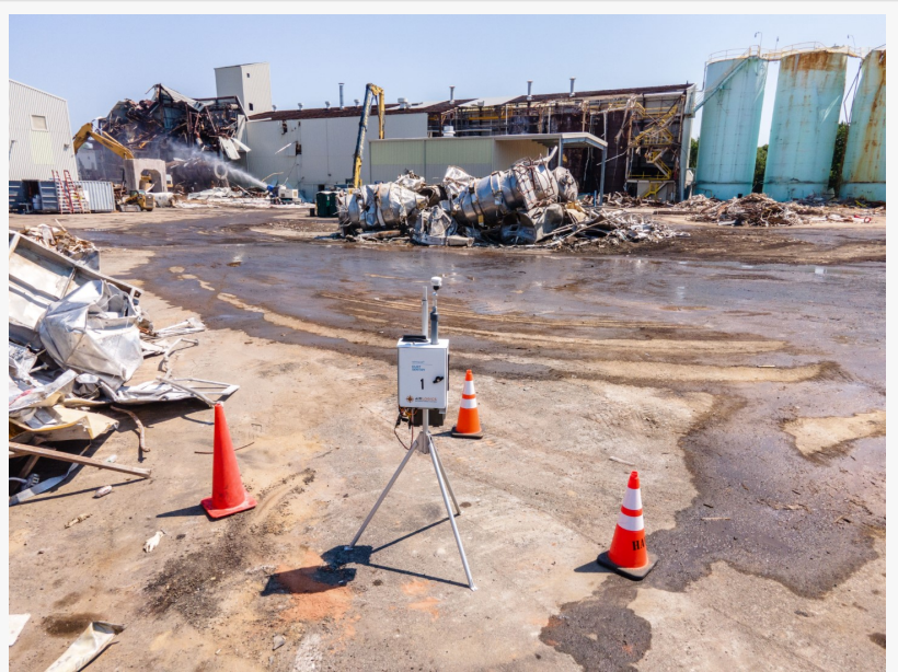
Perimeter Monitoring System
