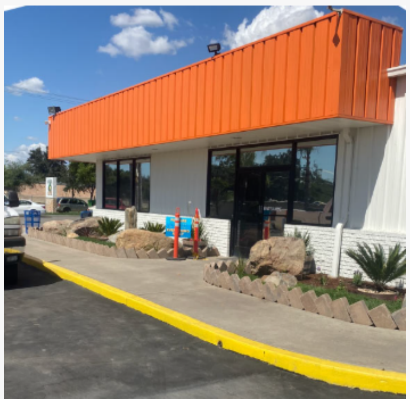
A commercial property exterior refreshed by Ponce's Quality Painting Inc., featuring durable protective coatings.
