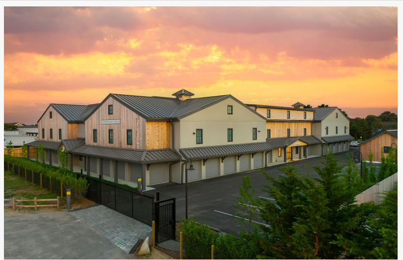
The 5-level storage facility includes covered parking. Photo by Patrick Coulie Photography
