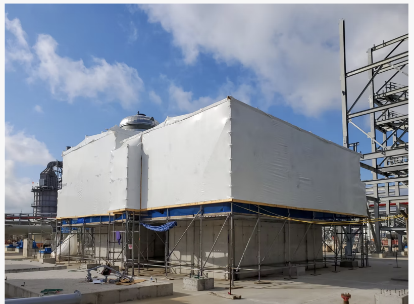
Oversized industrial module protected with custom industrial shrink wrap designed for large-scale projects, including data centers, modular construction and export applications.
