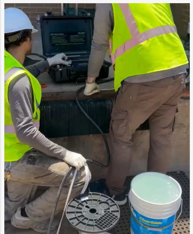
Sewer Camera Inspection
