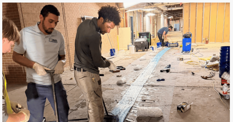
Pipe lining working in school
