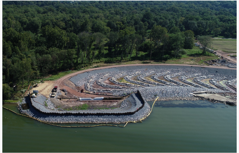
York Haven NLF Construction 2025
