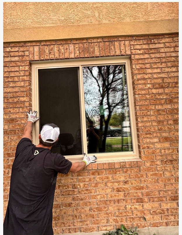
Elite Windows Team Replacing A Tucson Az Homes Windows
