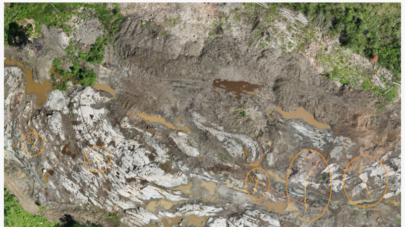
Zoomed in Detail of Stripped Area in Parbec's Open Pit Footprint with Channels in Orange
