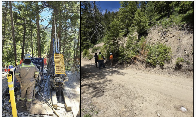
LEFT: Drilling Rig 03 (Left) at hole HH-GG26-004 on Ds10; RIGHT: Ds8 after drilling is completed. Three holes were drilled on Ds8 (HH-GG26-010, (HH-GG26-011, and (HH-GG26-012). Taking advance of the placing the drill sites on and very close to the access
