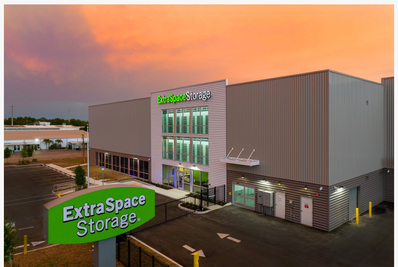
The 3-story, 96,843 NRSF development delivers 928 storage units to 2480 17th St. in Sarasota, FL.
