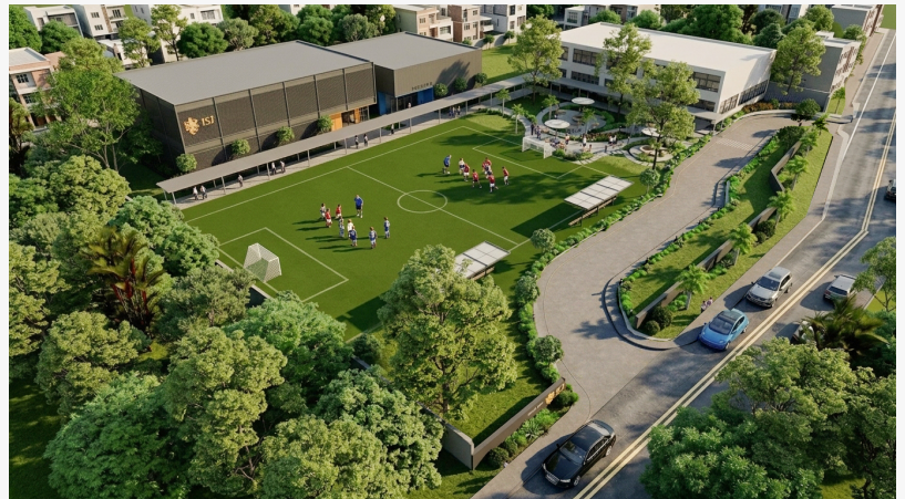
An aerial view of the new ISJ Senior Campus in Pondok Indah, South Jakarta, with its full-size football pitch, gymnasium, and classroom buildings. Opening 2028.
